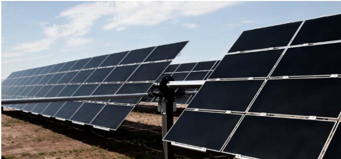
Plate 1. Example of a typical frameless solar array mounted on a single axis tracking system 8
